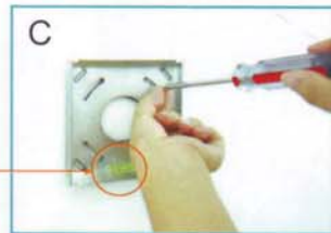
C Level the bracket to intend altitude, install the bracket on the wall.
